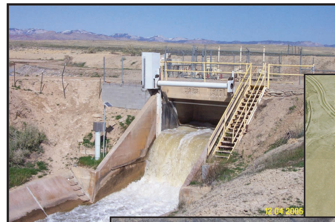
Automated turnout and pump station for reservoir
